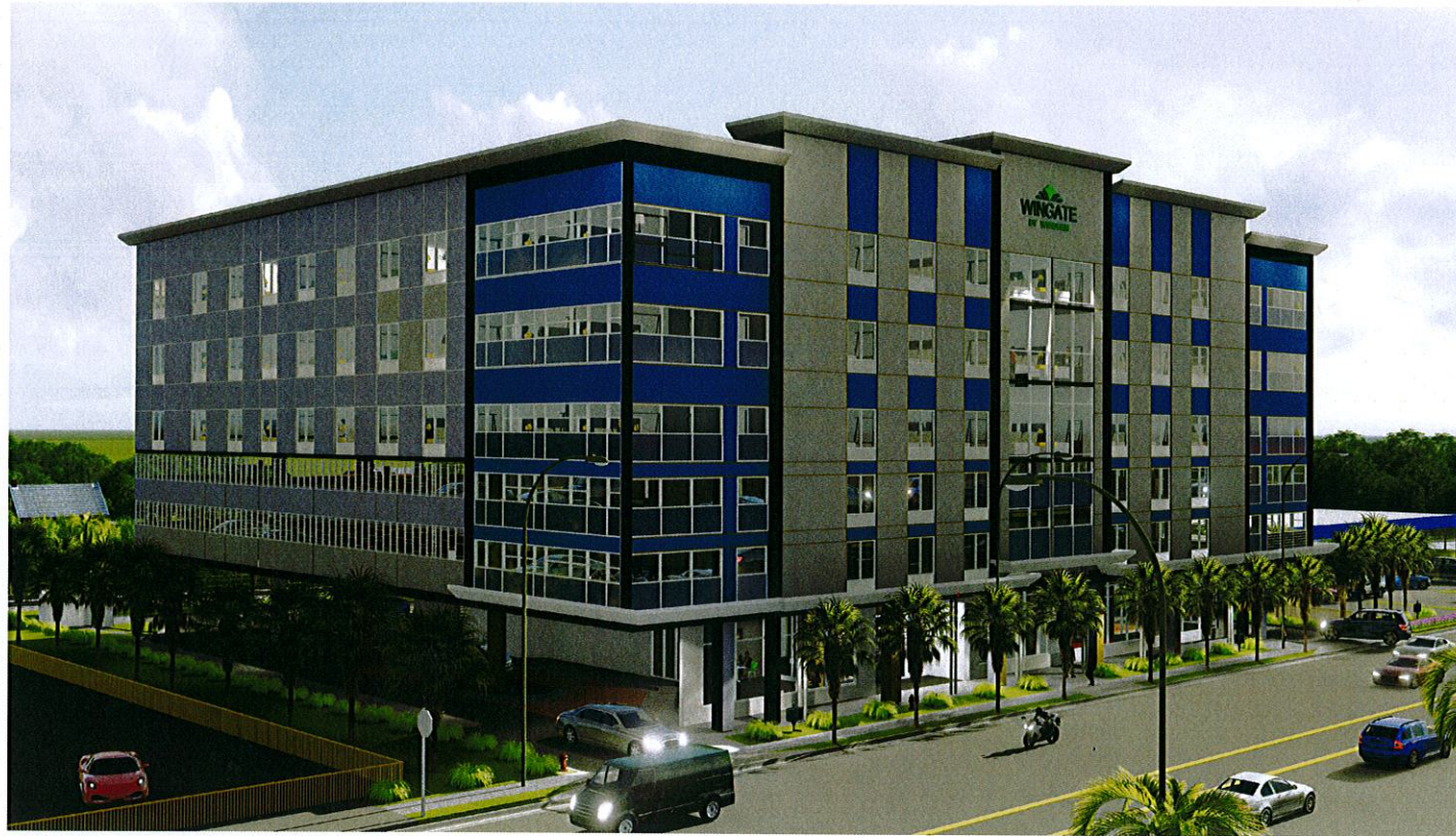
View from the South of North Federal Highway
