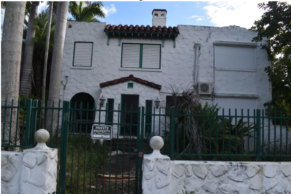
Street View looking southerly of northerly elevation
