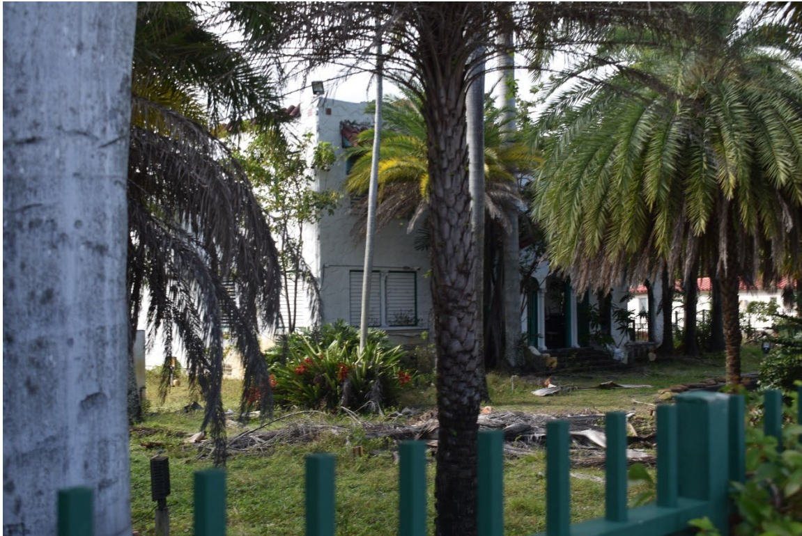
View looking northwesterly from S. Federal Highway
