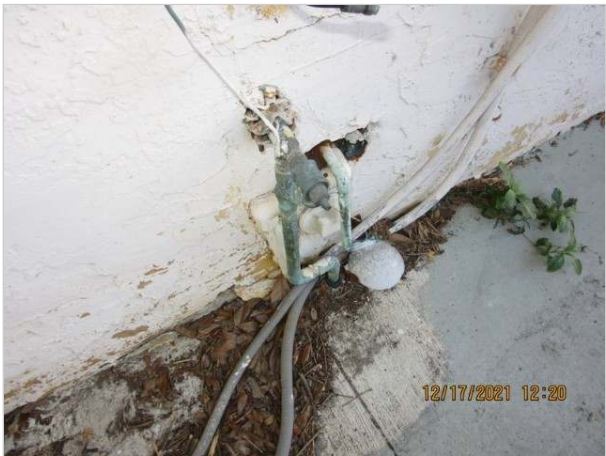
The meters and the supply wires had been removed.
