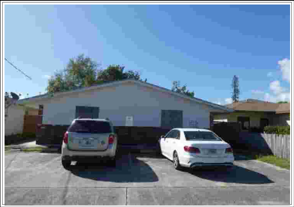
FRONT VIEW OF SUBJECT PROPERTY
