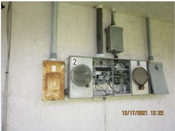
The meters and the supply wires had been removed.
