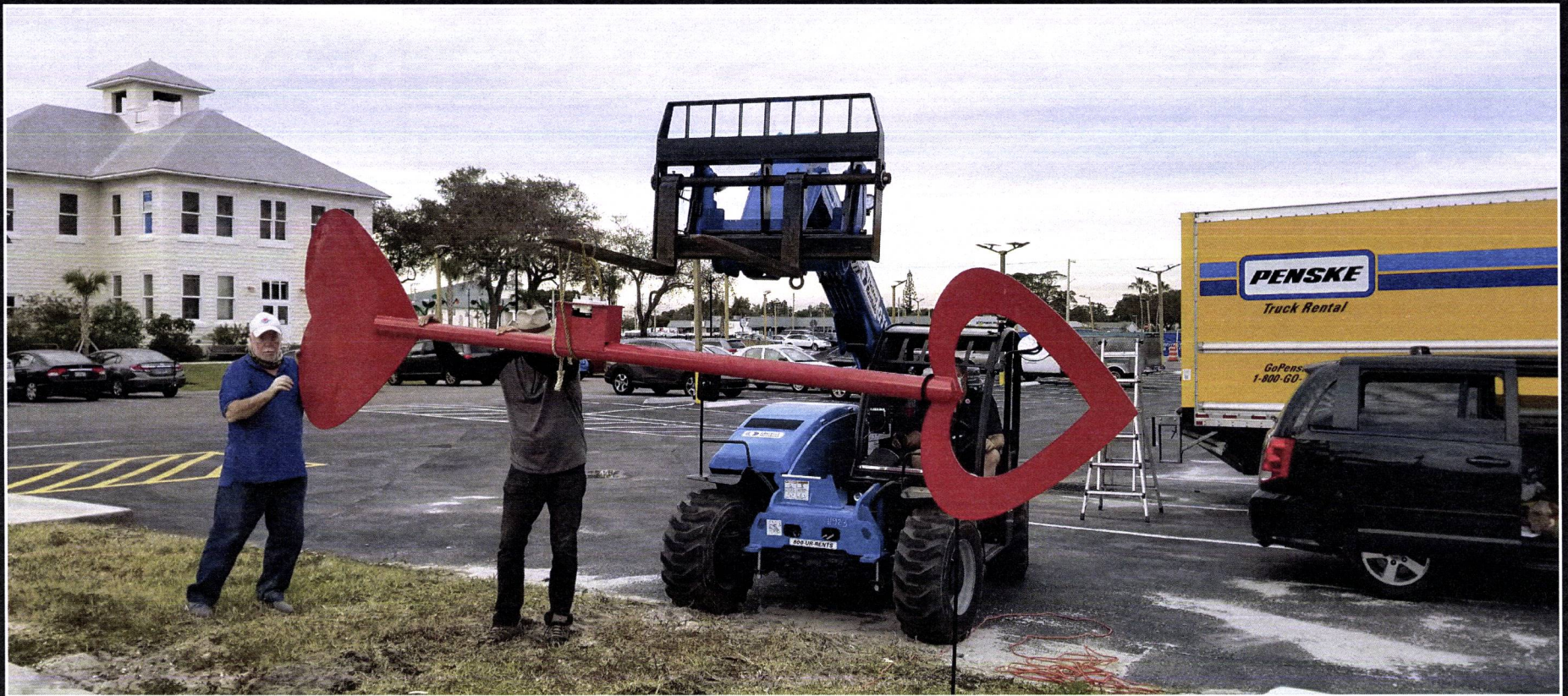
Installing the weathervane in Boynton Beach
