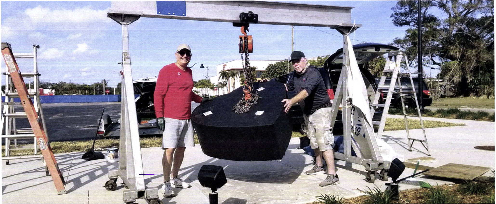
Moving the heart shaped concrete base which weighs 2,100 pounds
