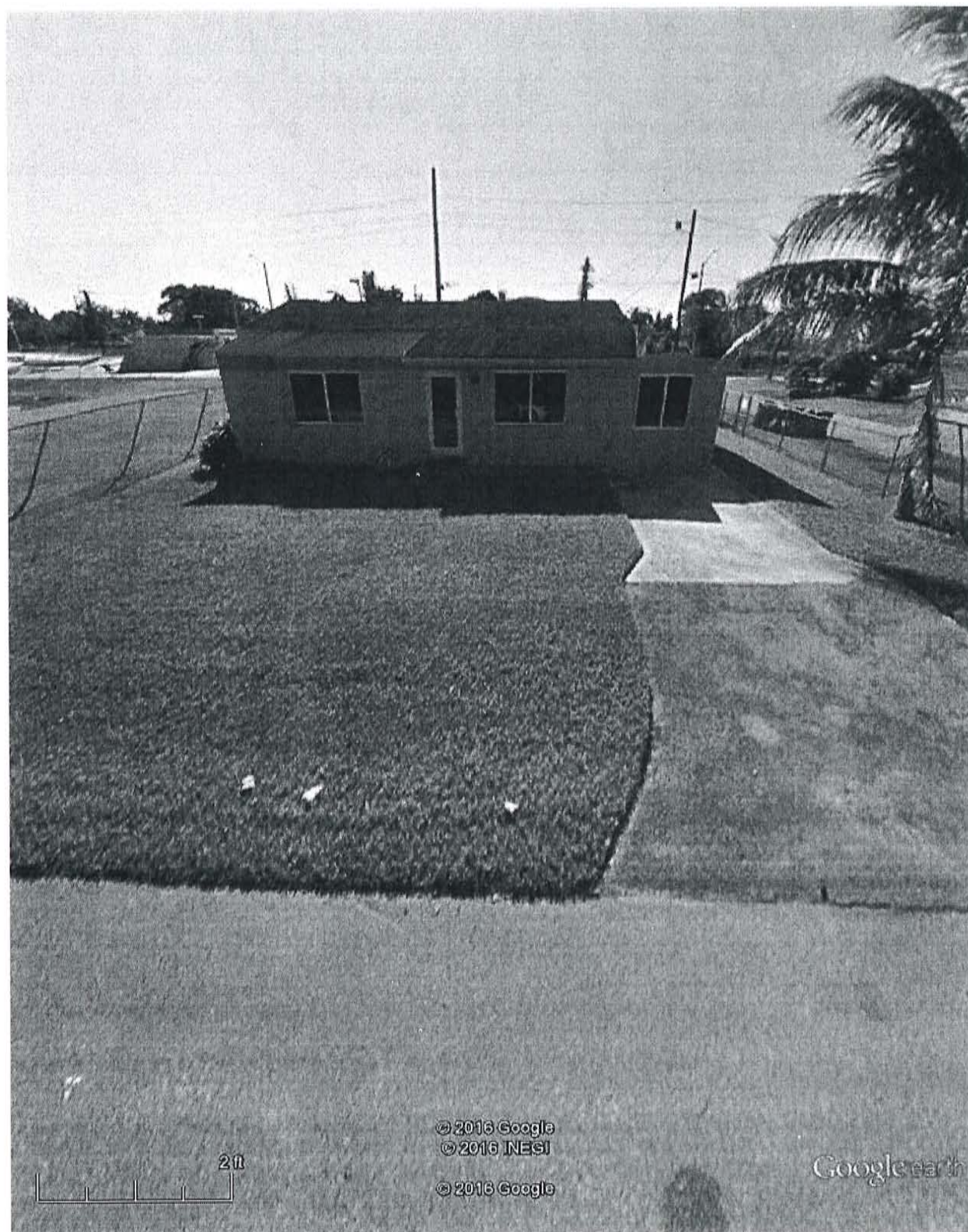
Front view of building
