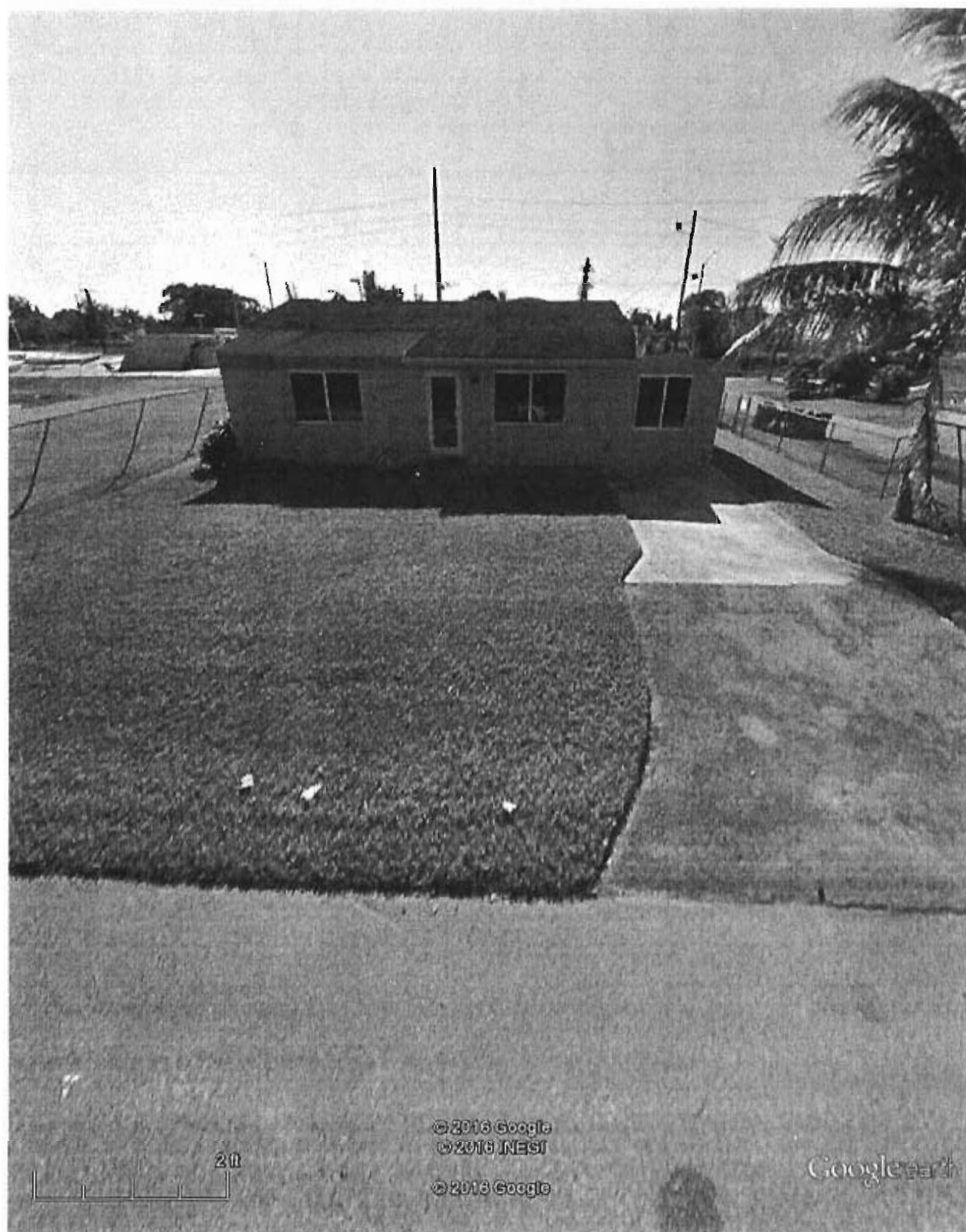
Front view of building
