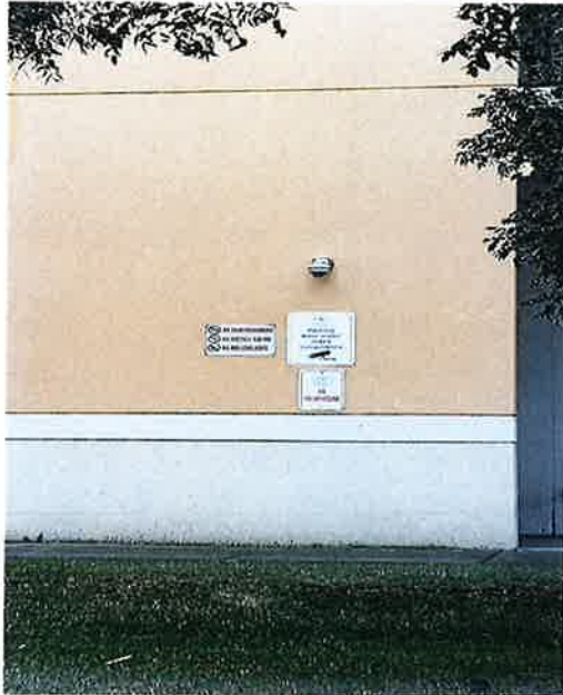
(Exterior of Parking Garage with Visible Signage posted)
