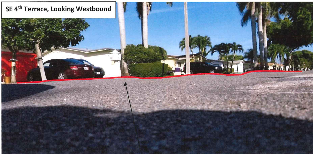
Figure 2 (Continued) – Photos – Dania Beach Southeast 4 th Terrace Road Reconstruction and Swale Project (Stormwater Resiliency) —Shows degraded pavement, crackling, “washboard” effect, and surface deterioration due to road subbase deterioration
