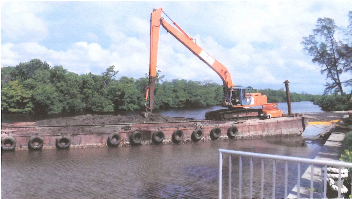
1. Eastern portion of the project site, facing northwest. Material being dredged mechanically from barge.
