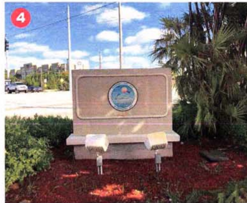
Southwest of intersection at Griffin Rd. & Anglers Ave. Remove foundation.
