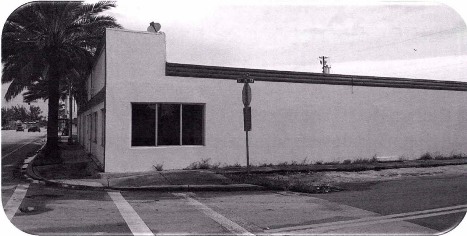
Facing northeast on S. Federal Hwy
