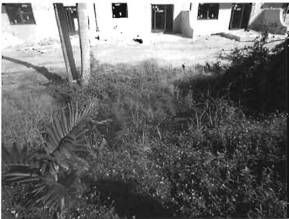
Photo 8. Drainage swale on northern portion of the property.
