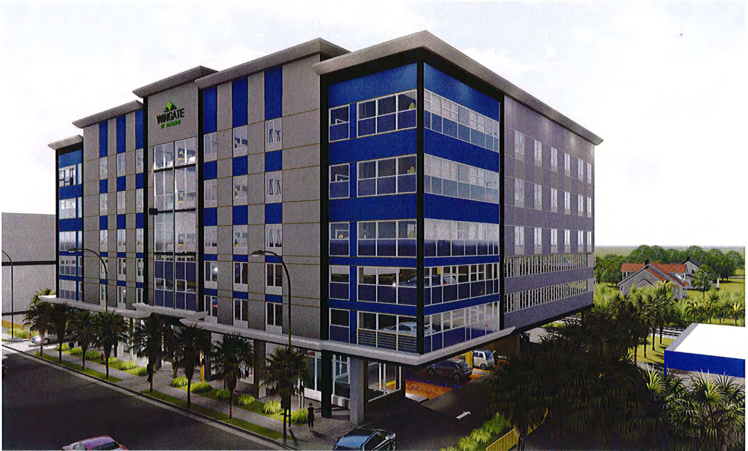
View from the North of North Federal Highway
